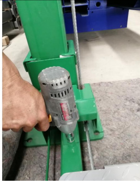
Conection way of lock release bar for manual lock release type
